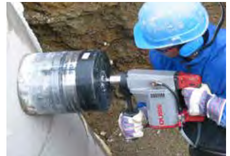
DRILLING IN A CONCRETE SHAFT – wet, hand-held
