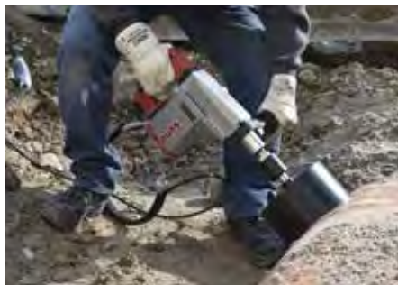
DRILLING IN A PLASTIC PIPE – dry, hand-held
