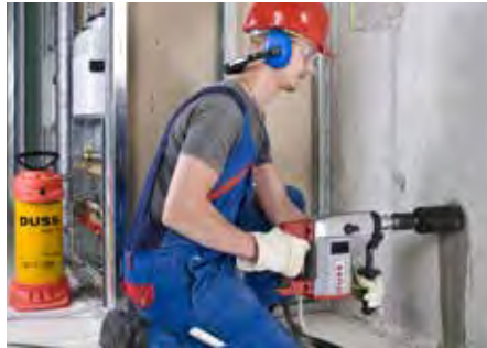
ELECTRICAL SOCKET SINKING in concrete – wet, hand-held
