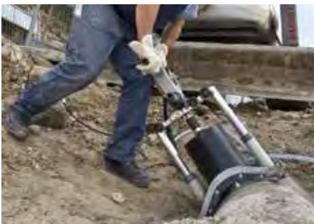
DRILLING IN A CONCRETE PIPE – wet, with BST drill stand
