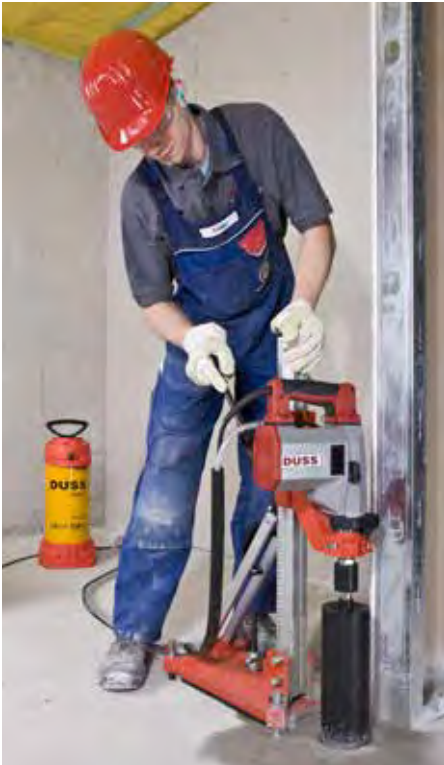
WET DRILLING in concrete – with BS drill stand
