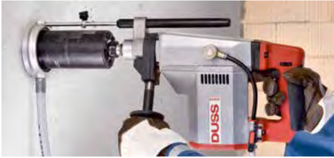
Wet socket sinking in concrete with water extraction
