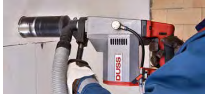
Dry socket sinking in sand-lime brick with dust extraction
